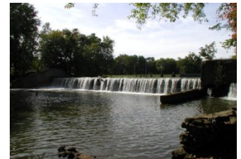
Newton Falls Dam
